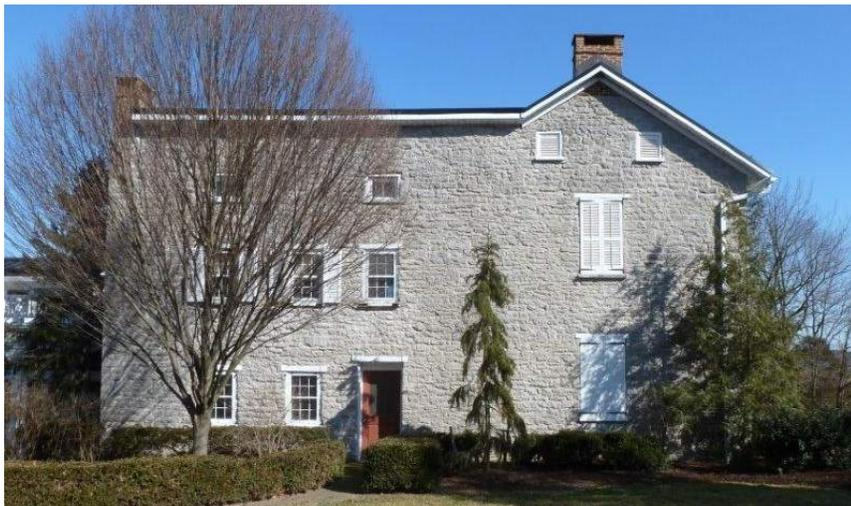
**Figure 23** The kitchen wing extending in back of the Thomas<sup>IV</sup> Barber house has a shed roof rather than the typical gable roof, providing a third floor of back bedrooms tucked under the sloping eaves. Closed false shutters that give the impression of windows below the chimney are a curious original feature of the house.
