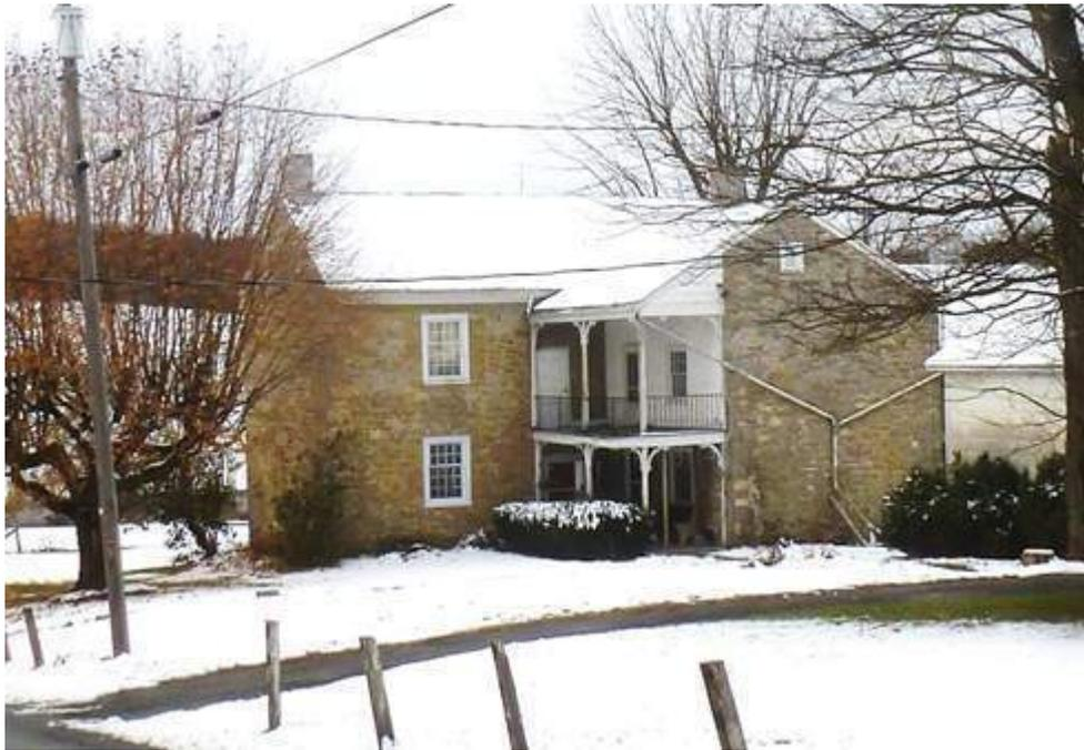
**Figure 30** Back of the Clingan House showing stone kitchen with two story porch. The rear of the Thomas<sup>IV</sup> Barber house has been extensively altered and added on to, but it probably had a covered porch at the ground floor, and possibly a two-story porch similar to this one on its rear wing.
