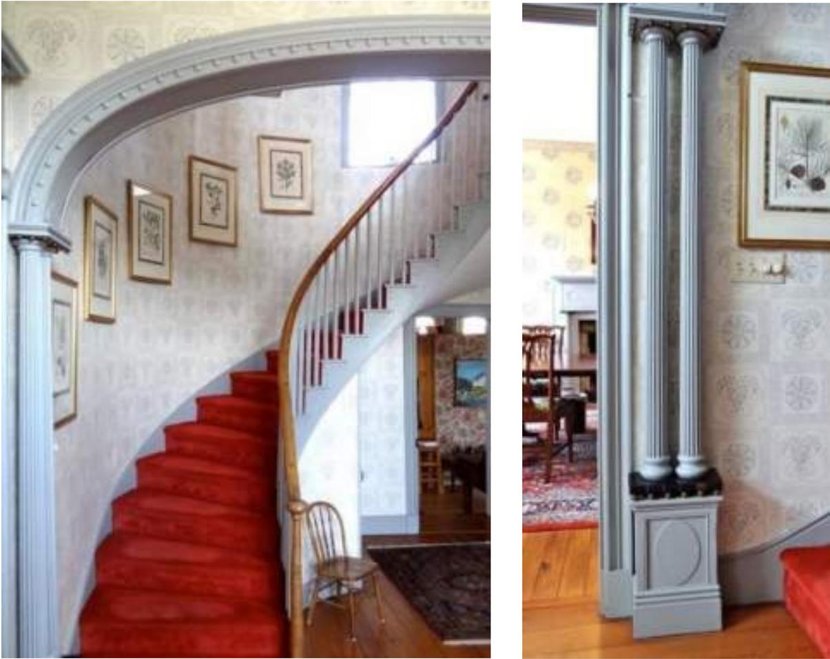
**Figure 24** Entrance hall of the Thomas<sup>IV</sup> Barber house with spiral staircase and elliptical archway. The double columns which support the archway rest on a carved wood ledger book.
