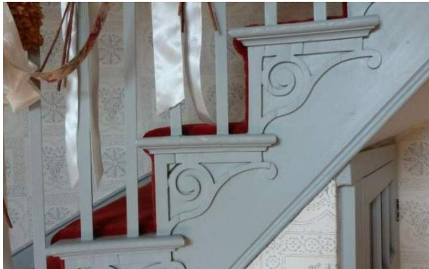
**Figure 32** Step bracket trim of circular stair in the Thomas<sup>IV</sup> Barber house, based on builder's manual.
